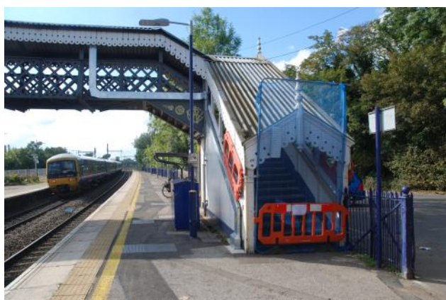
No way over the old footbridge
