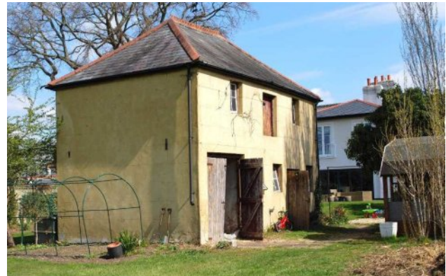
Old Coach House behind Cranford House on Boundary Road
